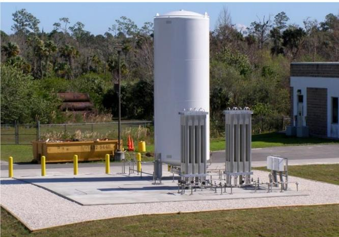
New 9,000 gallon Liquid Oxygen Tank for the Surface Water Treatment Plant at the Dyal WTP.
