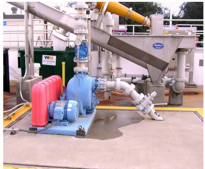
New grit pump and grit classifier. The new grit pump sits atop the filled in vault where the old recessed-impeller pump was housed.
