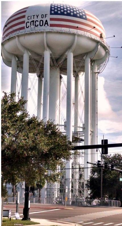
Scaffolding is going up under the elevated tank in preparation for sand blasting and painting.
