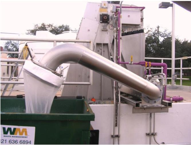
New bar screen, conveyor belt and washer/compactor unit.
